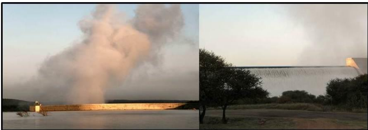
Figure 1.2: The dam wall of Flag Boshielo Dam
