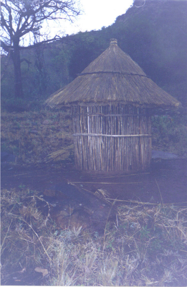
Figure 3: Wall made up of poles
