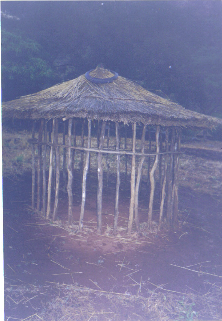
Figure 2: Poles fitted in holes to form a wall structure
