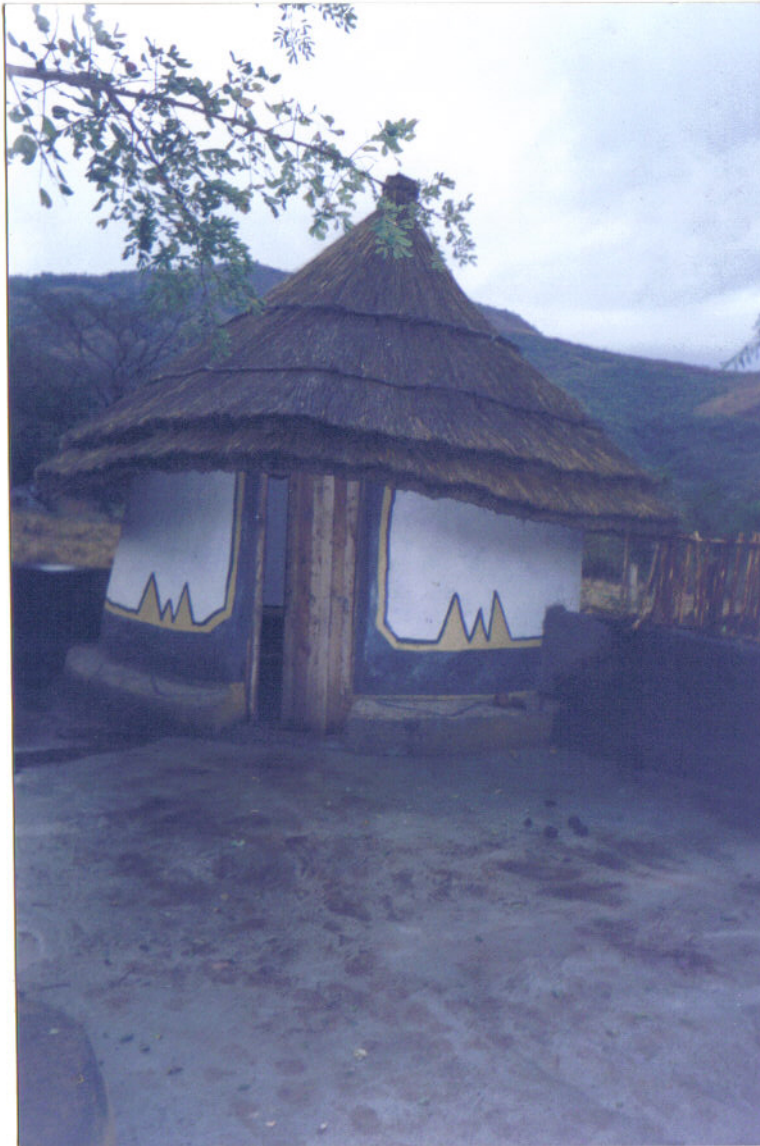
Figure 8: Bapedi's decorated roofing
