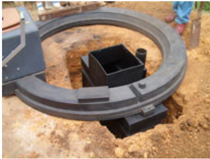
Place housing and pedestal over sump
