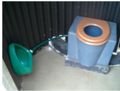
Erect hut around pedestal and attach urinal
