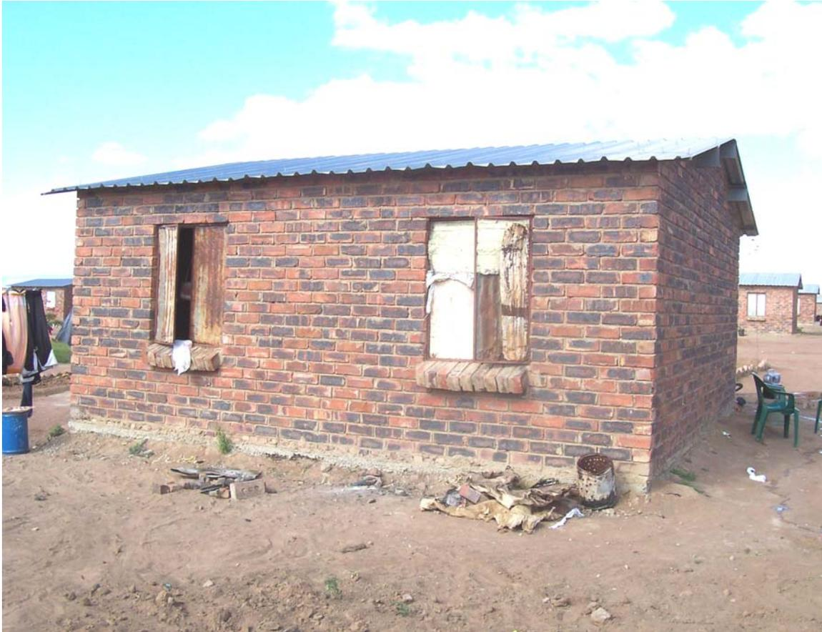
**C4.** This roof was blown off by the wind and the walls collapsed because of the poor quality of materials and workmanship.
