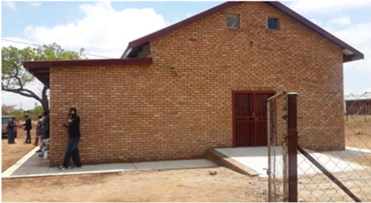
Annexure 3: Premises of Sekwena Art and Craft Project at Mohodi Ha-Manthata
