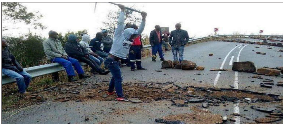
Figure 1: Protesters Dig up Tarred KZN Road as Service Delivery Frustrations Spill Over
