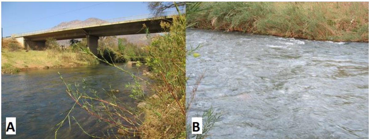
Figure 2.9: Site 4 (A+B), Burgersfort Bridge.
