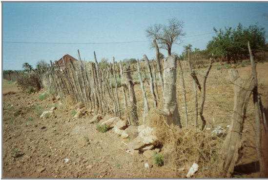
Figure 4.9 Fencing. The mean number of poles used to fence a yard of approximately 25 m 2 and the sizes required are indicated in Tables 4.4A and 4.4B.
