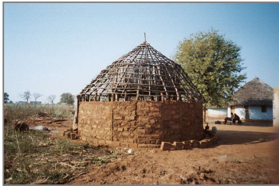
Figure 4.7 A kitchen and a maize grain store within the roof. The radius of a kitchen is approximately 2.6 m from the centre. The mean number of poles and the sizes required to construct a kitchen and the inside maize grain store are indicated in Tables 4.4A and 4.4B.
