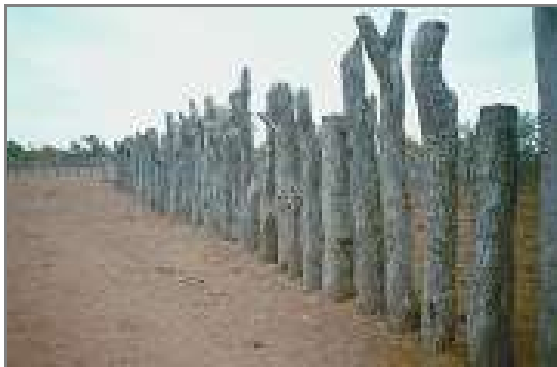
Figure 4.10 A medium to large sized cattle kraal. The size of the kraals ranges from about 5 m 2 to 15 m 2 , but some are not absolute square. The mean number of inserted poles in the soil and the sizes required to construct a cattle kraal are indicated in Tables 4.4A and 4.4B.
