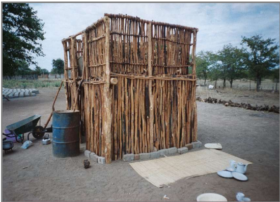
Figure 4.6 A traditional maize grain store. The size of outside grain stores sampled is between 2.4 and 2.5 m 2 . The mean number of poles and sizes required to construct an outside maize grain store are indicated in Tables 4.4A and 4.4B.
