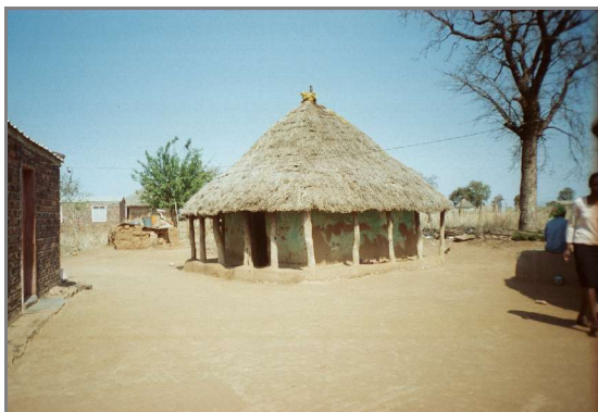
Figure 4.8 A traditional hut. The radius of the hut is approximately 3 m. The mean number of poles and sizes required to construct a hut are indicated in Tables 4.4A and 4.4B.
