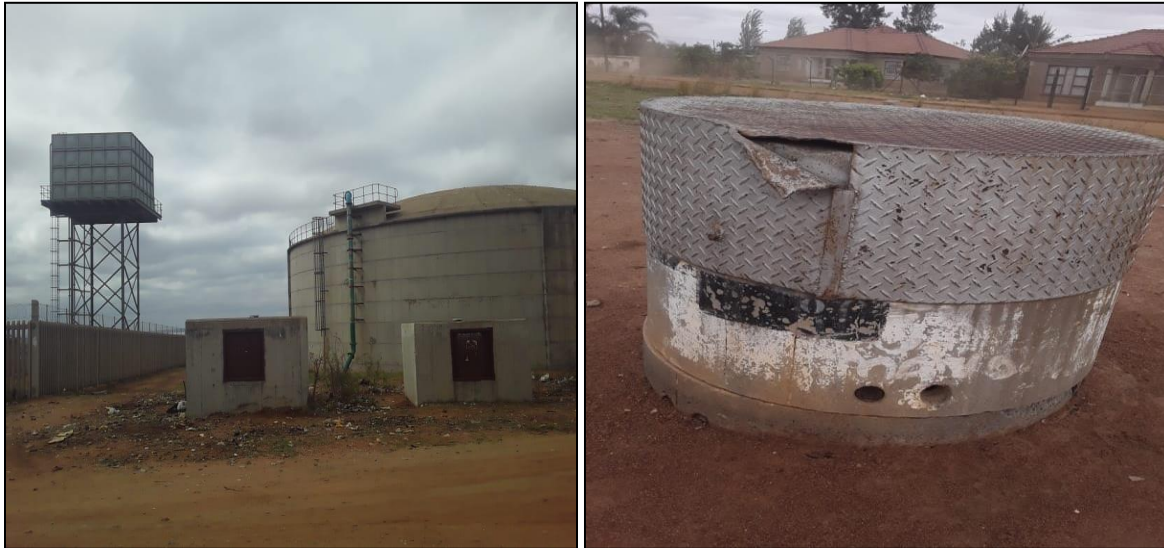
Figure 4.9: Some of water infrastructures situated at Ga-Thoka village.
