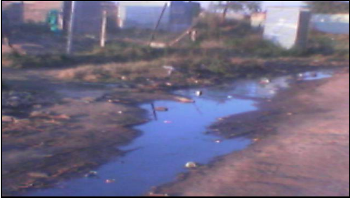
Figure 21: Situation after raining condition
