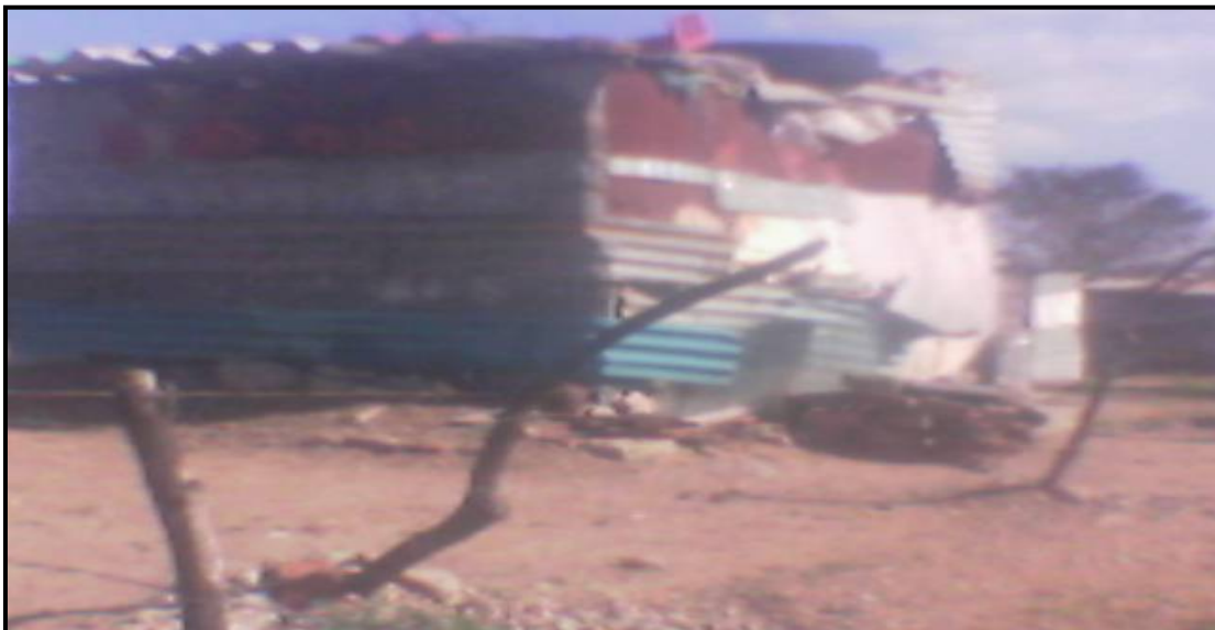
Figure 6: Shack built from steel
