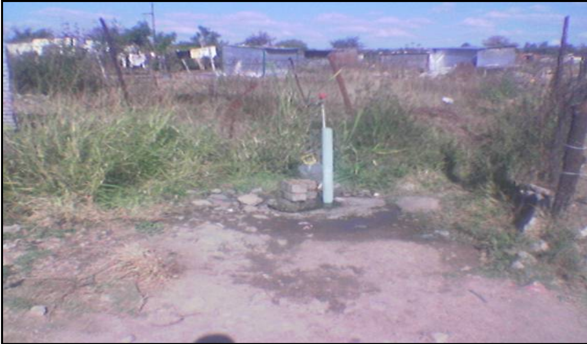
Figure 26: Street standpipe for water collection
