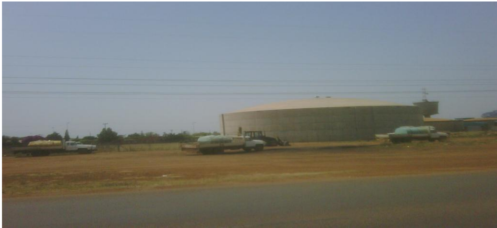
Figure 3: Bulk Water Supply Reservoir in Themba with Trucks collecting water for the un-serviced areas in the part of North East region
