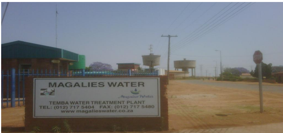
Figure 4: Waste water treatment plant in Themba Area (North East) servicing the population
