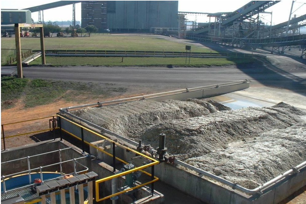
Figure 2.6 Typical limestone neutralization plant (courtesy J P Maree)
