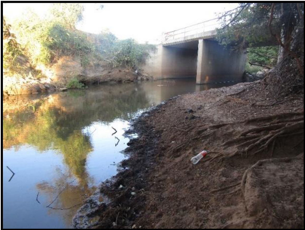
Figure 2.10: Site 8 is situated downstream of the bridge that leads to Adelaide Police Station of the Nwanedi River. Image taken during summer survey.
